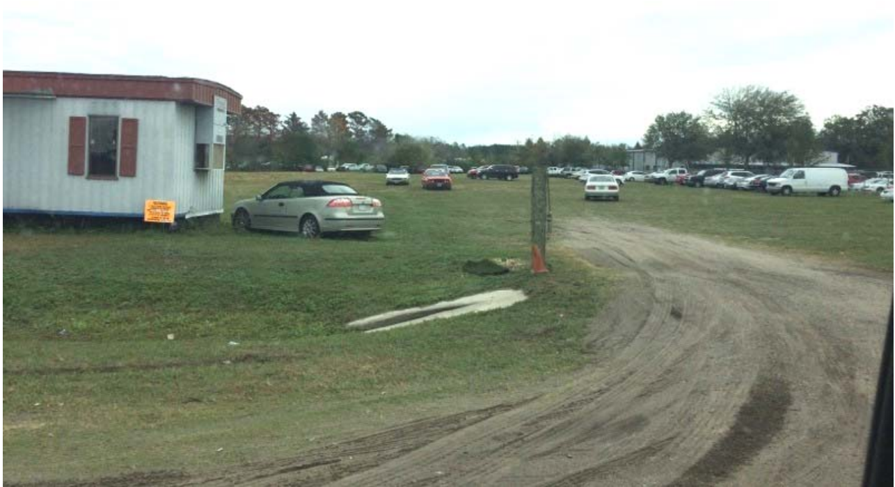
The subject site facing east from Kings Rd. (US 1)
