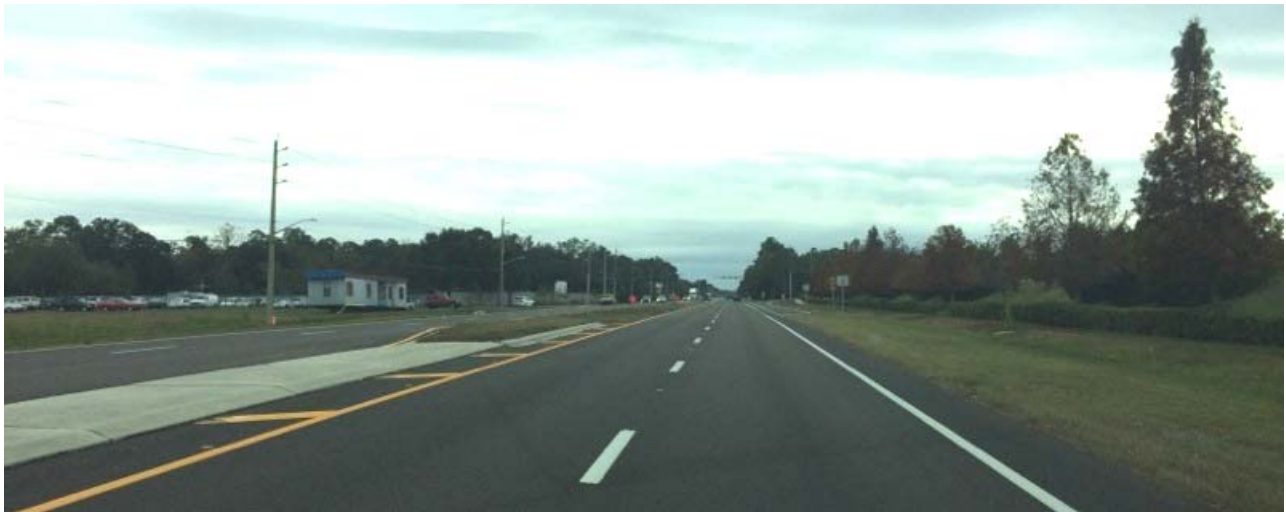
The subject site on the left facing north along Kings Rd. (US 1)
